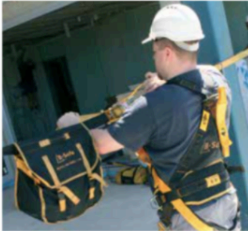
Web temporary life line, ratchet tensioning method.
