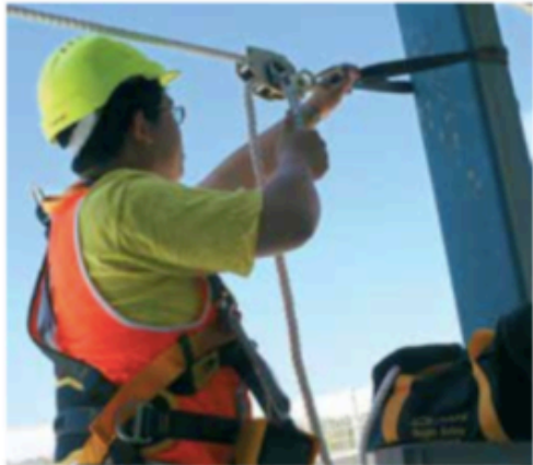
Rope temporary life line being installed and tensioned.
