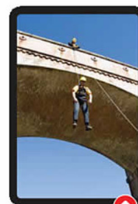
Suspended person without S/A Lanyard
