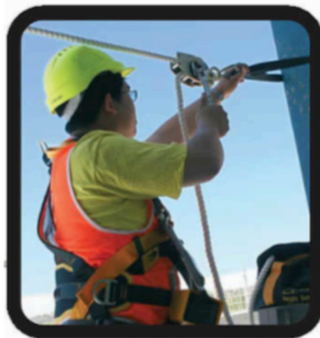
Rope temporary life line being installed and tensioned.
